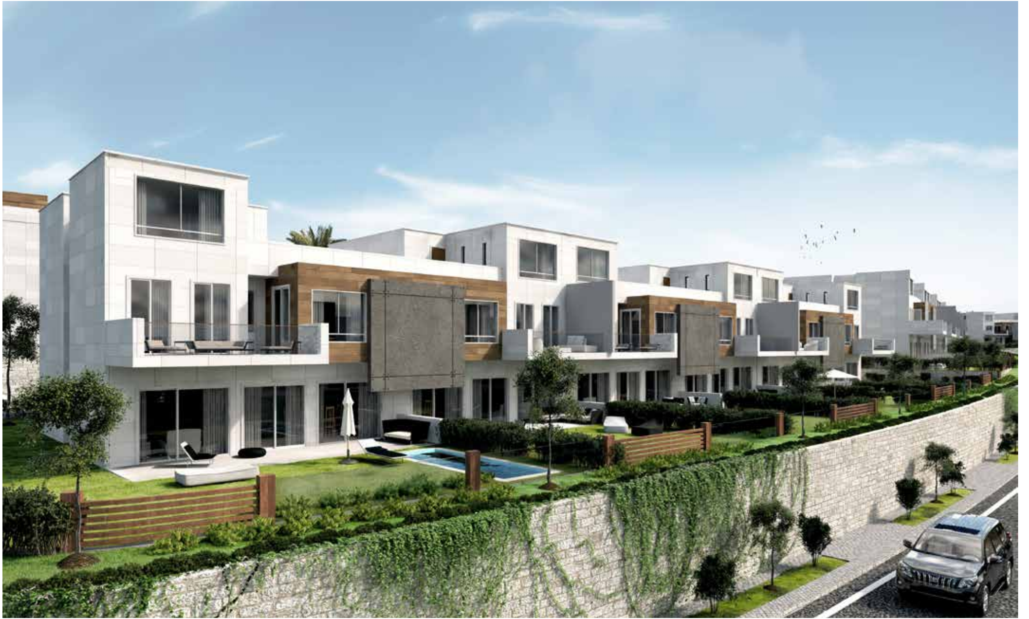
Building G Townhouses / Back View
