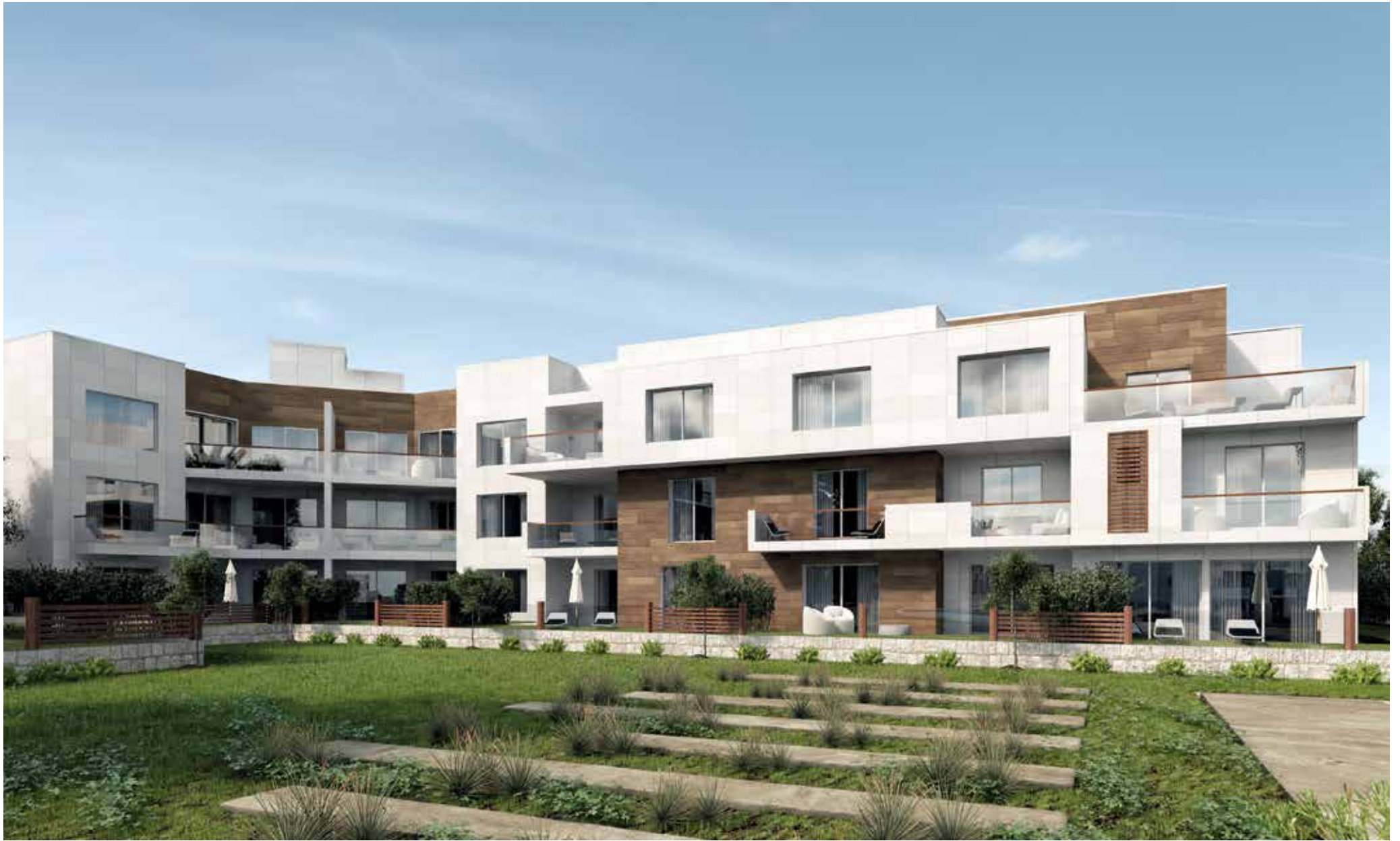
Building F Apartments / Back View
