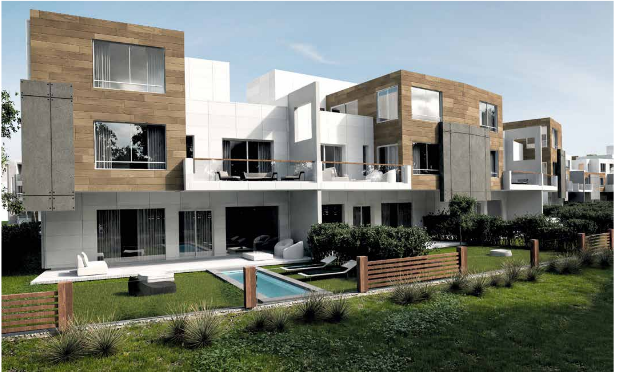
Building J Townhouses / Back View
