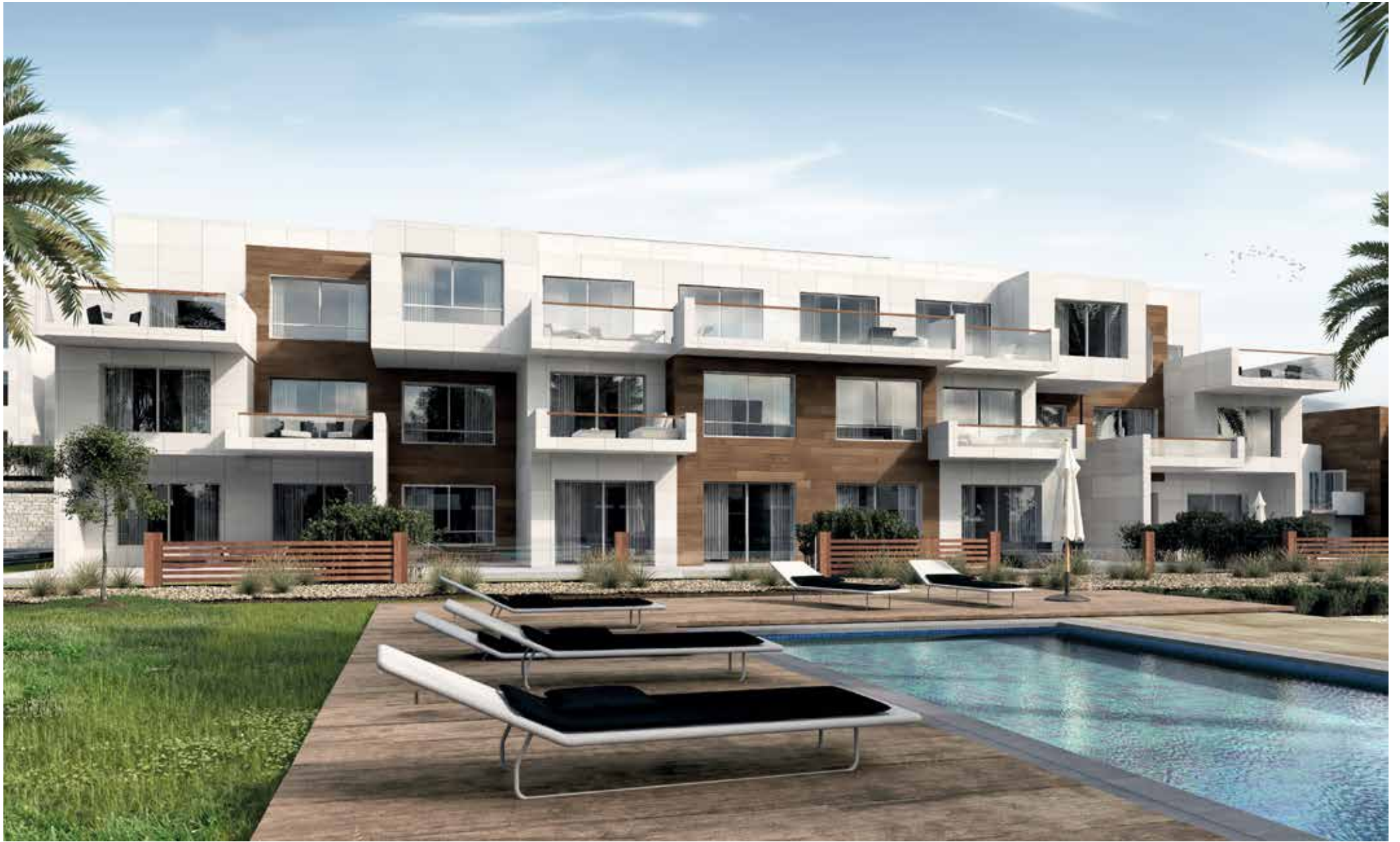
Building A Apartments / Back View
