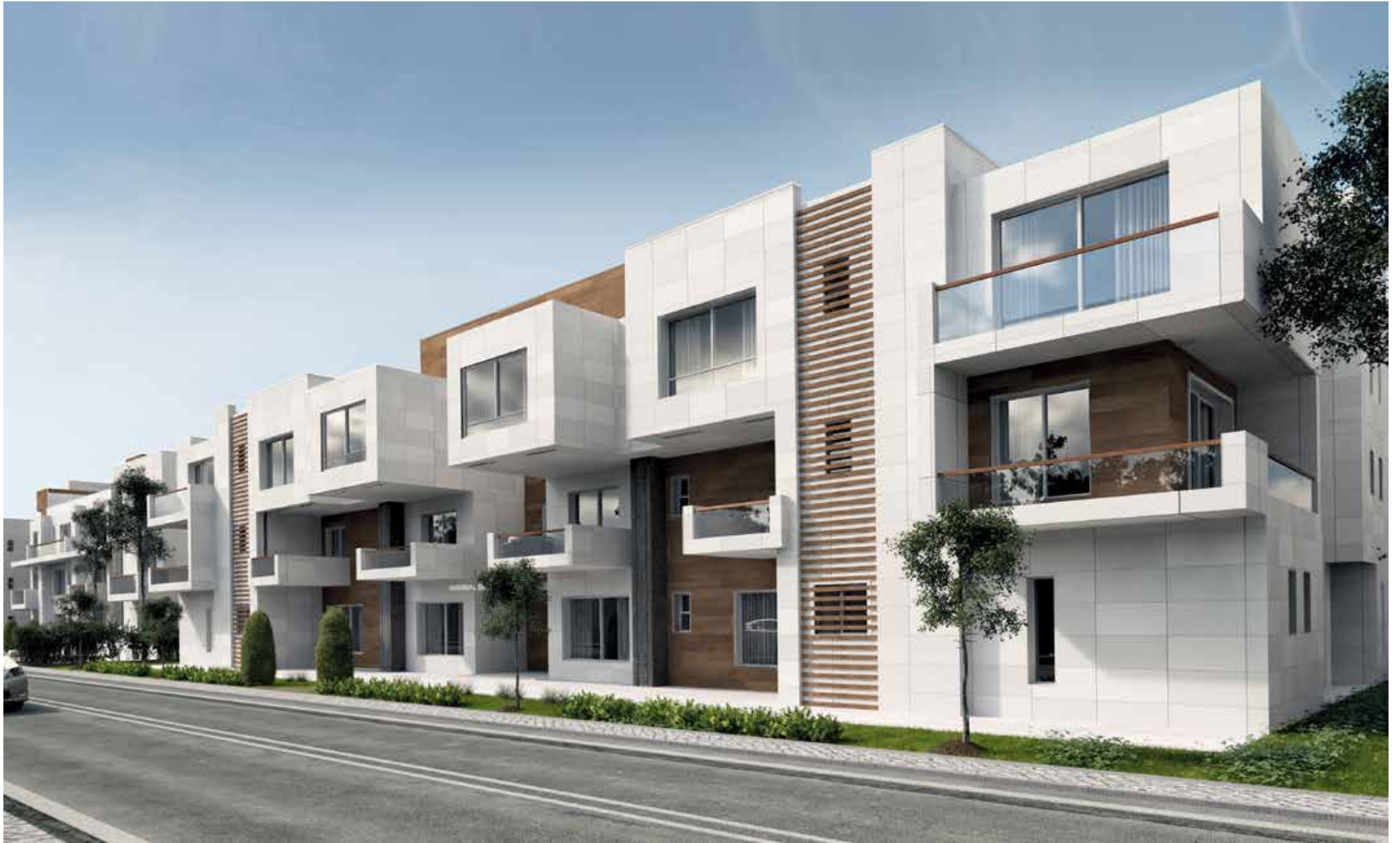
Building A Apartments / Front View
