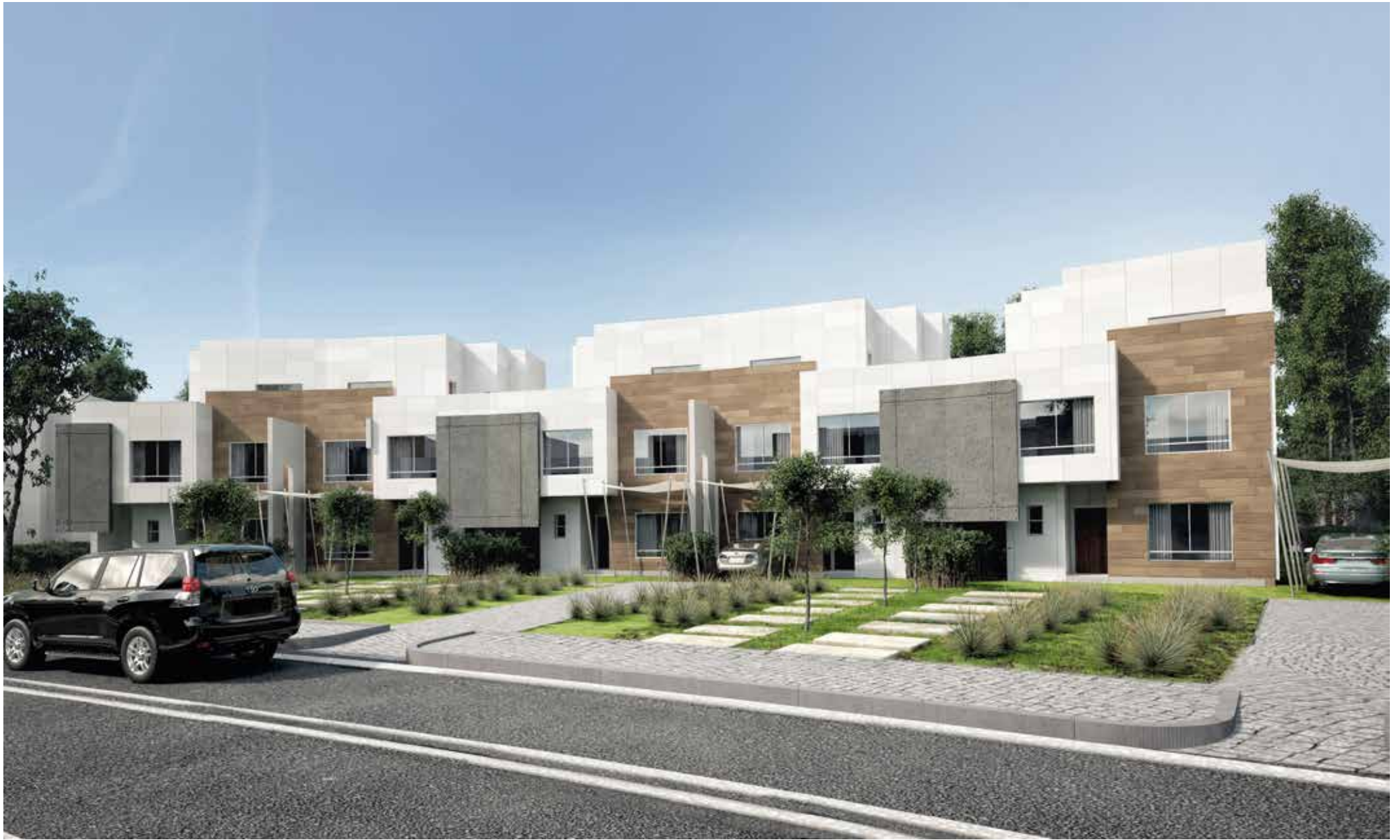
Building J Townhouses/ Front View
